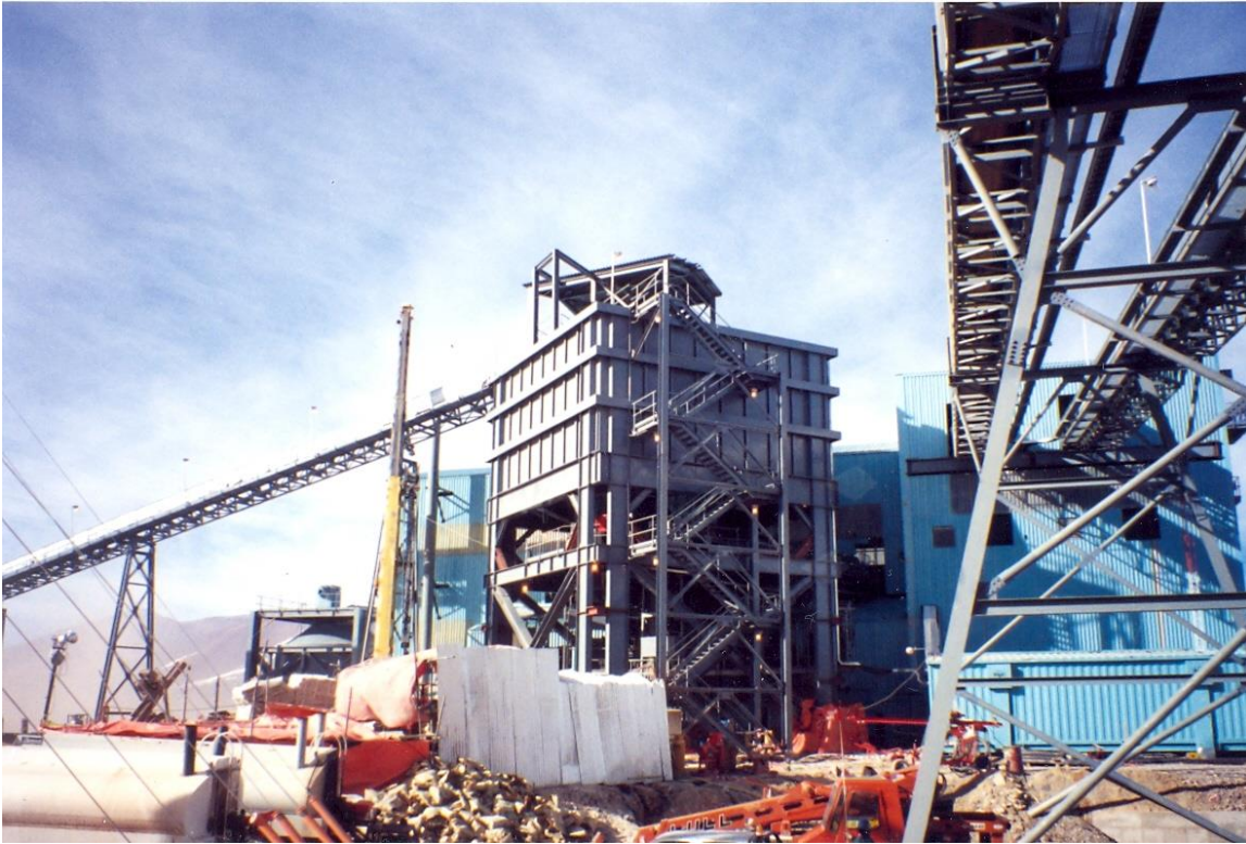
Looking South At The Recirculation Bin, Stairway & Conveyors Note the two W36x135 columns at each corner
