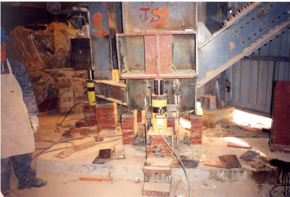
Looking At Corner C From The Outside
