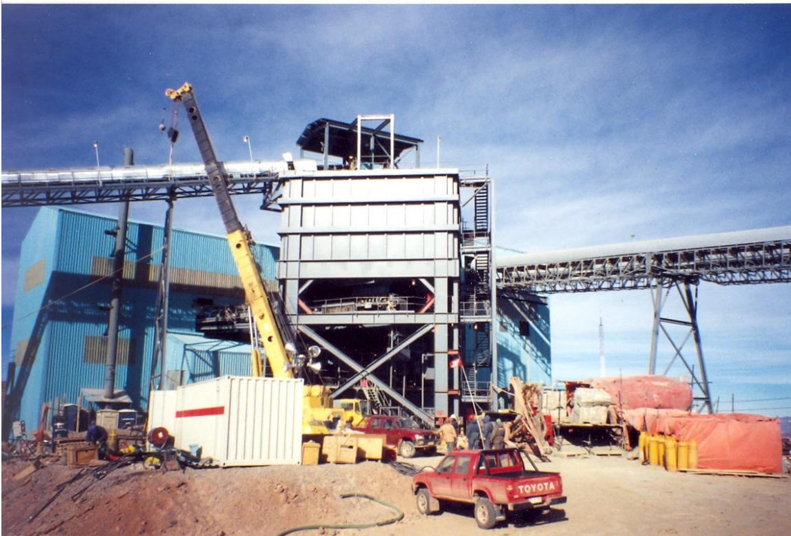
Looking Southwest At The Recirculation Bin, Stairway & Conveyors
